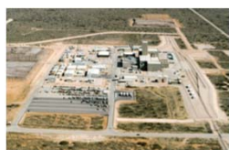
WIPP Surface Facilities
